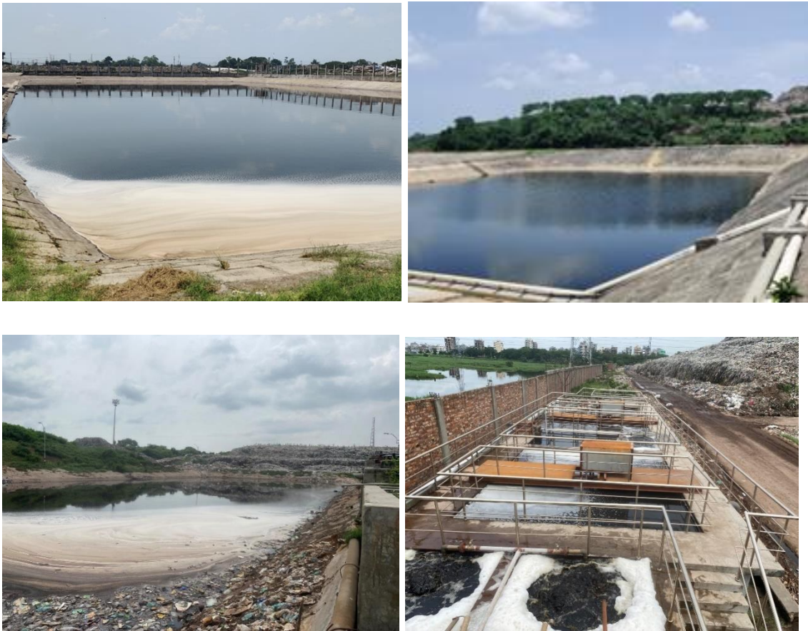
Fig 6: Raw and treated leachate collection from raw and treated leachate ponds at Aminbazar and Matuail Landfills
